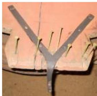
I believe this was a replacement bracket because the holes in the front where the nails are located are showing the holes. There was originally a flat piece of metal with a hook instead of a Y shape with hook.
